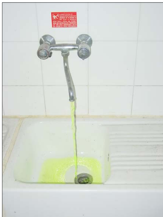
Figure 4 Fluorescein diffusion in water system
